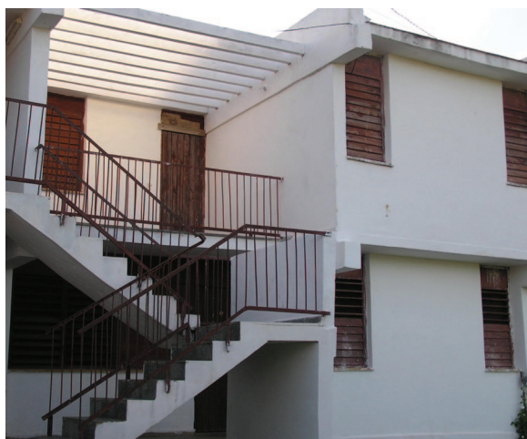
Figure 1. Exterior of typical consultorio (primary care clinic).
